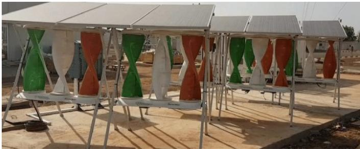
In Bamako, Mali, MINUSMA has made a small-scale investment in pilot technology that combines wind energy and solar energy. It consists of six vertical axis wind turbines and three photovoltaic (PV) panels. Power generation works at wind speeds between 2 and 18.5 m/s and temperatures from -30 to 50 °C. The electricity, 9 kW capacity, is fed directly into the battery bank to provide a back-up system for basic ICT energy requirements.
