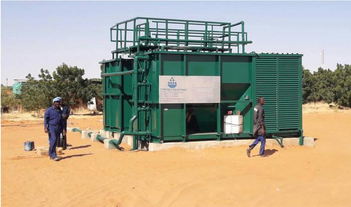
In South Sudan, UNMISS purchased 39 wastewater treatment plants between 2014 and 2016. Starting in 2017, the mission started reusing the treated effluents (i.e. wastewater recycling) for water-consuming activities such as dust control, washing of vehicles and cleaning generators, and landscaping and gardening. In doing so, UNMISS has reduced clean water consumption throughout the mission and realized a cost saving of USD 11,970 per year.
