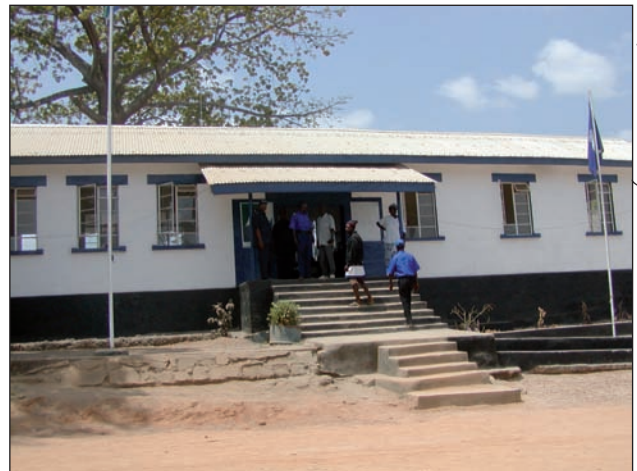
Newly renovated police station in Koidu
