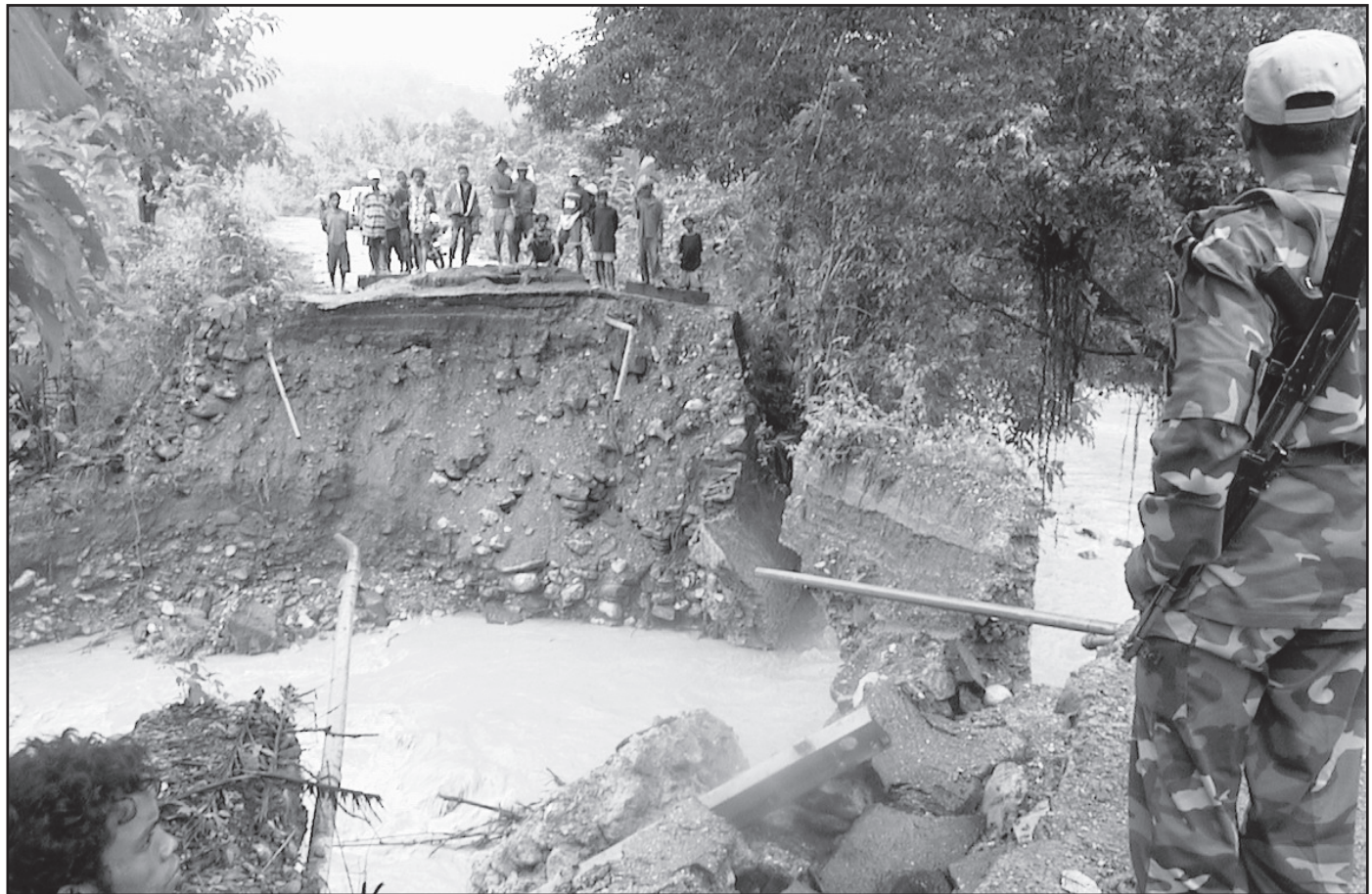
Populasaun Viqueque brani hamrik iha udan laran besik ponti. Mota lori ponti, halo kotu dalan iha distritu husi fatin seluk iha rai laran. Injeneiru Forsa Paz husi batalhaun Baglades halo ona ponti neebe bele tahan to tinan 50. Hanesan mos kompanhia konstrusaun Australia nian halo hela projektu rehabilitasaun dalan iha reziaun neba nian, neebe estabiliza tiha ona atu hatutan fatin sira iha Viqueque laran .
